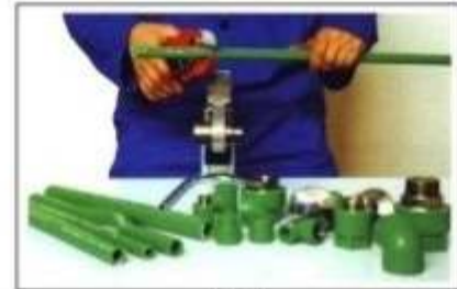
Fig.1 Cut required length with cutter
